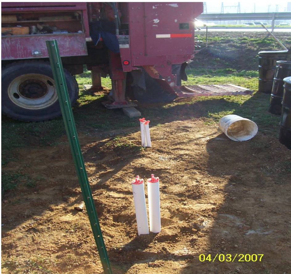
Photograph 2 – Air rotary drilling rig drilling monitoring well cluster PZ-E15.
