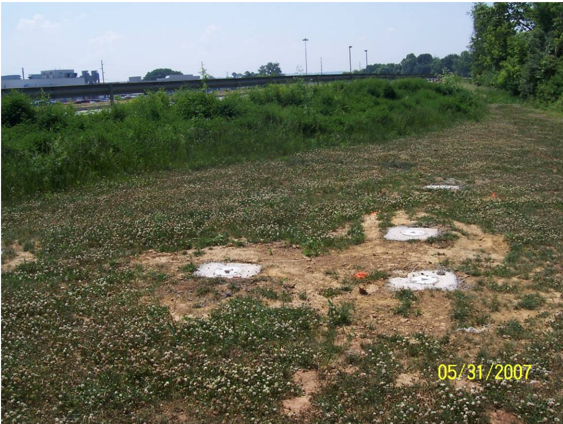
Photograph 12 – Completed SVE wells with drive-over covers.
